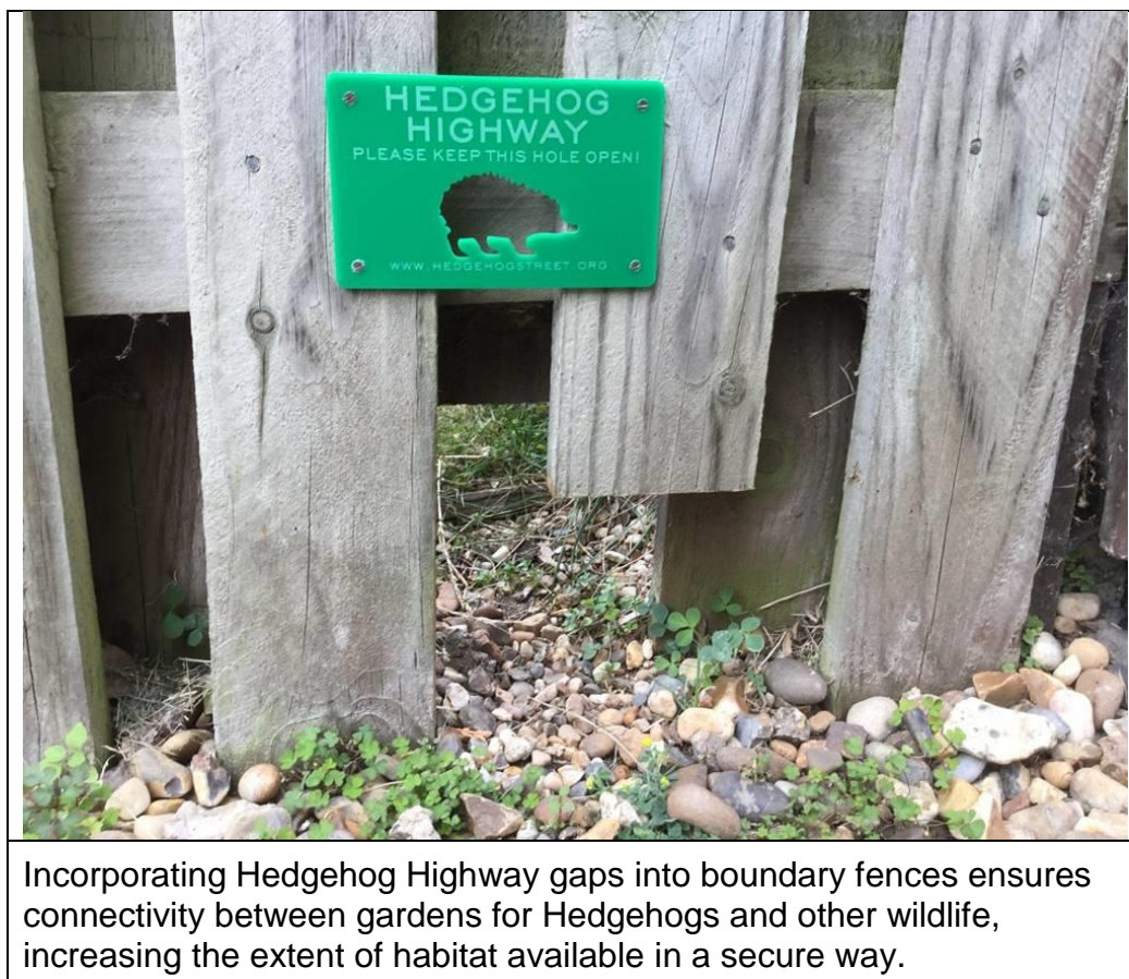
Figure 7 Hedgehog Highway gaps in boundary fence.
