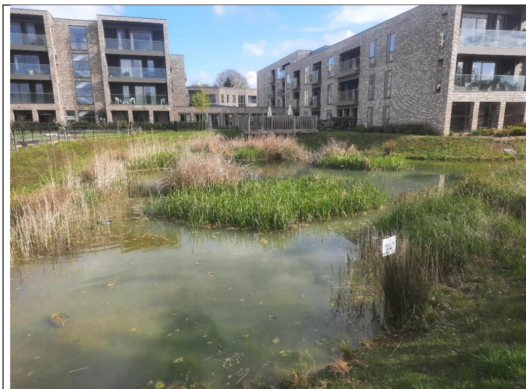
SuDS features should be designed to provide natural habitats appropriate to the surrounding landscape, using locally native species and managed to combine functionality and opportunities for biodiversity
