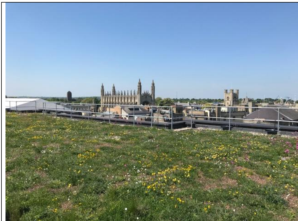
A biodiverse roof, showing a diversity of flowering plants in an open grassland structure. Habitat design and species mixes should reflect local conditions and stated conservation objectives
